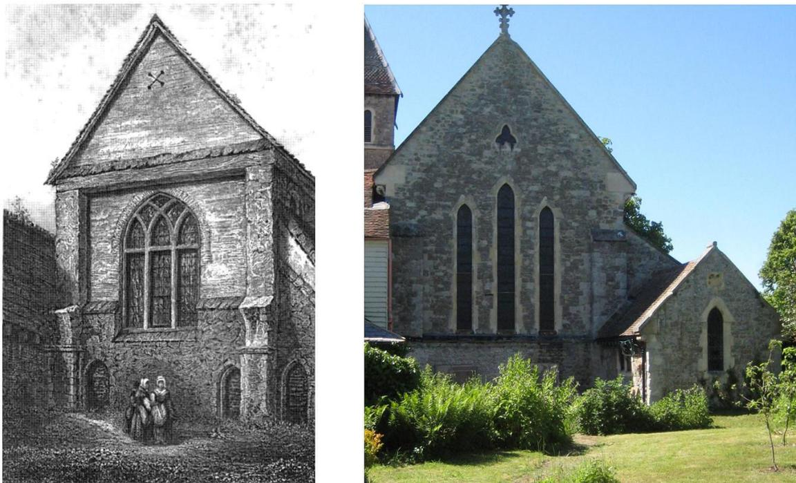
**Fig 7: Rear elevation of the east end of the Priory/Parish Church in 1845<sup>27</sup> and 2010, demonstrating Willement's rebuild. Note the aisle doors (now blocked) and the new vestry on the right.**
