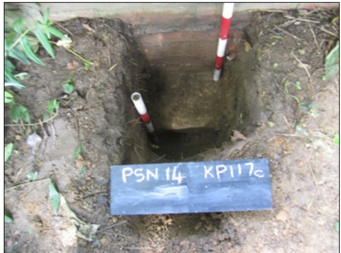
Fig 14: The finished pit, showing the concrete foundation.
