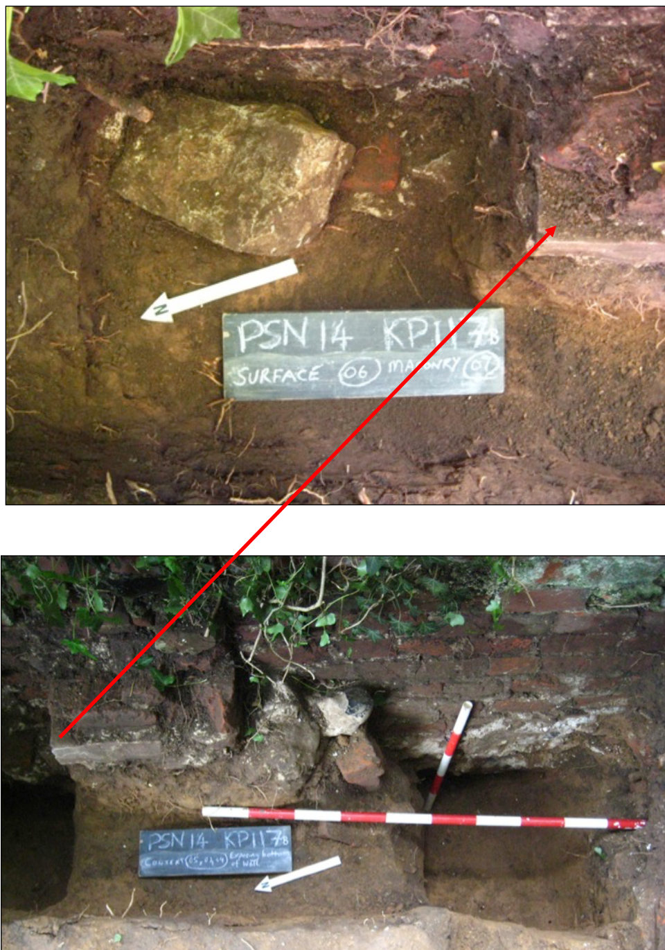
Fig 13: End stage. In the southern extension, the heavily mortared base of the wall can clearly be seen. In fact the wall just above this is quite 'snotty' (i.e. not pointed, lots of mortar dribbles) therefore not meant to be exposed to public gaze.
