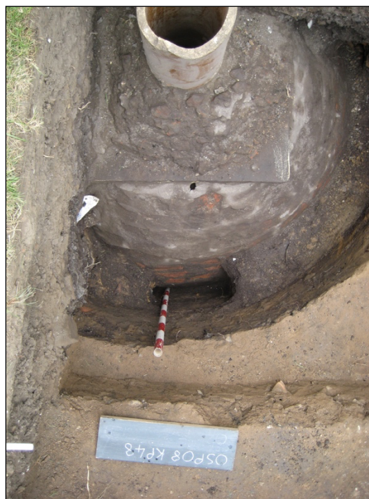
(b) Outside. Note the different phases. The access trench has been emptied and a slot taken down to reveal the brickwork.
